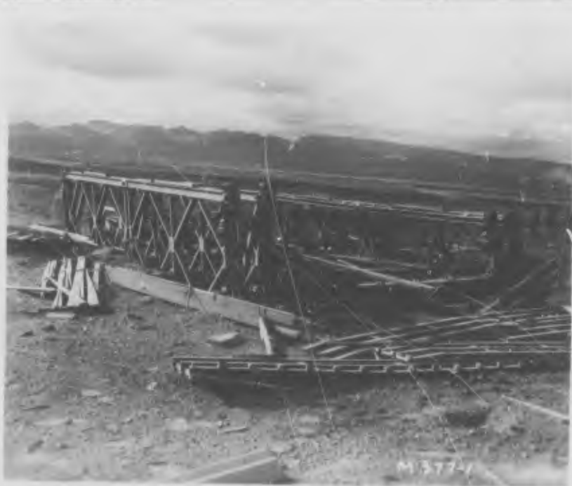
Bailey Bridge Before ↗ After ↘ Moved Sideways 5 Yards
